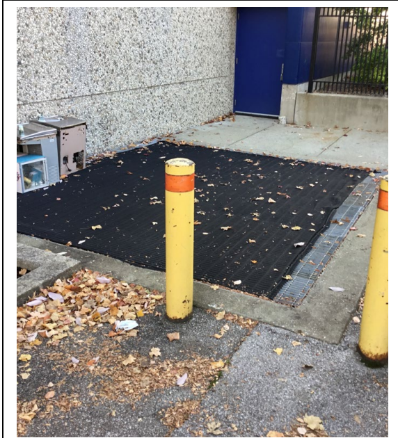
Figure 005 – Areaway access from above
