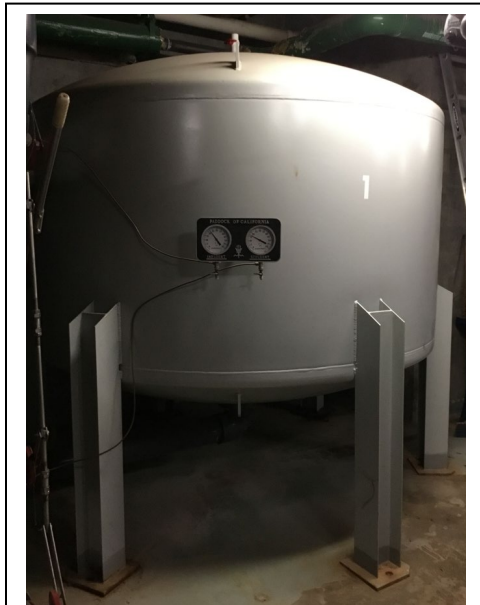
Figure 002 – Existing tank (typical)
