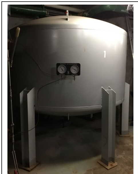
Figure 002 – Existing tank (typical)
