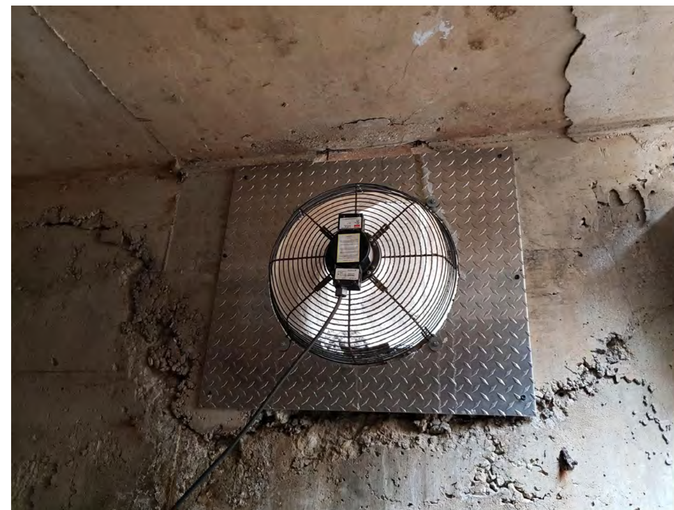
VIEW OF EXISTING EXHAUST FAN AND VENT AN EXISTING EXHAUST FAN WAS OBSERVED NEXT TO THE MANHOLE OPENING OF THE EXISTING VAULT. REMOVING EXISTING TOP SLAB AND INSTALLING NEW SLAB REQUIRES MODIFICATION OF THE EXISTING OPENING AND LOWER THE EXISTING FAN (SEE MECH DWGS).
