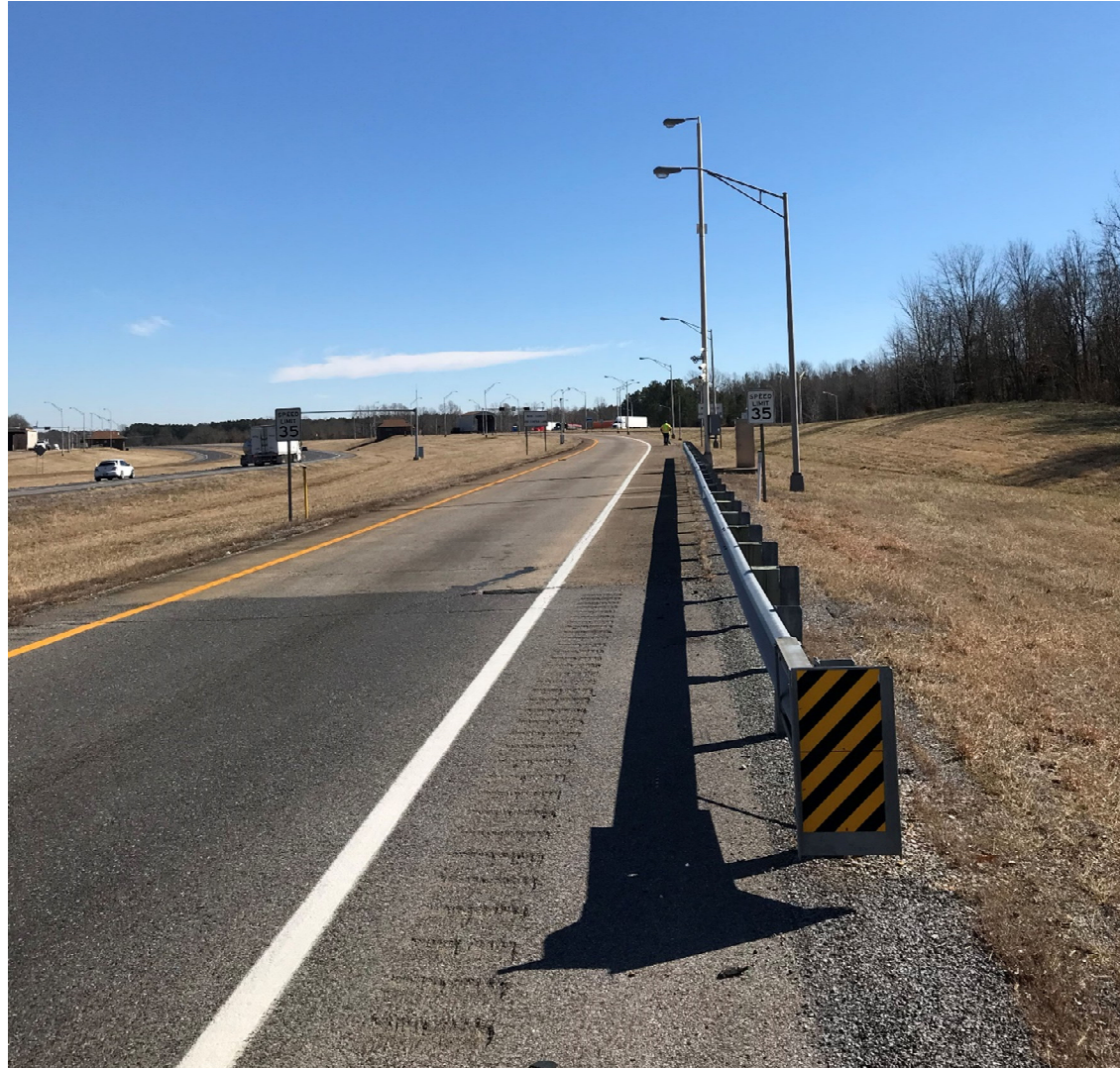
Figure 4. Start of Guardrail at KATS Camera Pole
