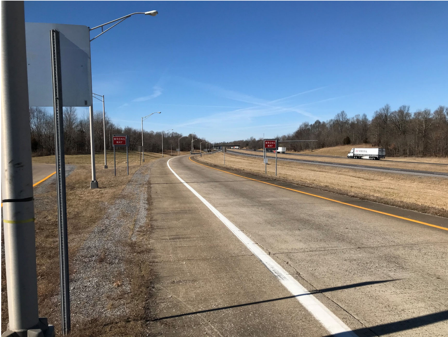
Figure 8. Ramp View toward Entrance
