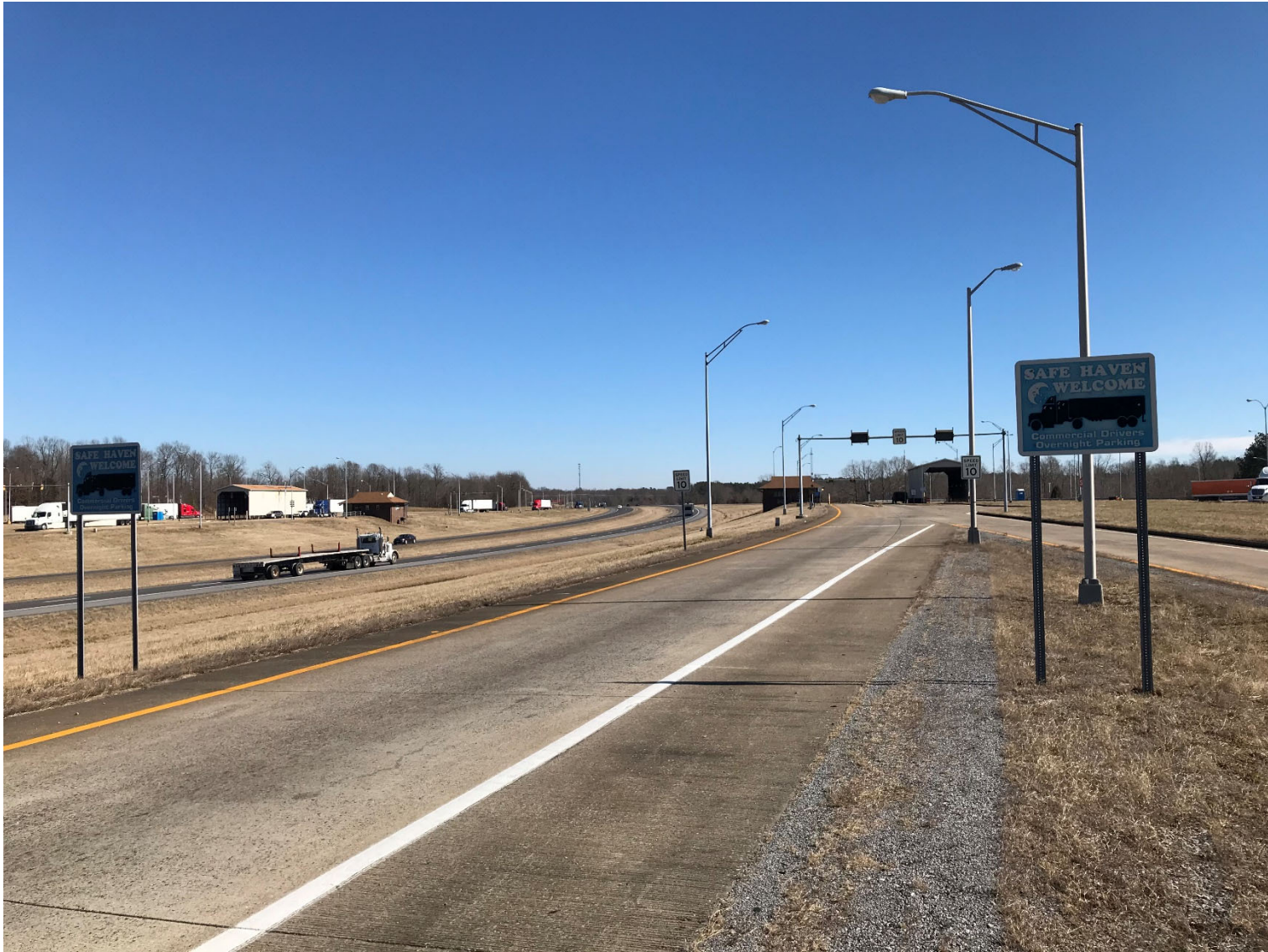
Figure 9. Ramp View toward Facility
