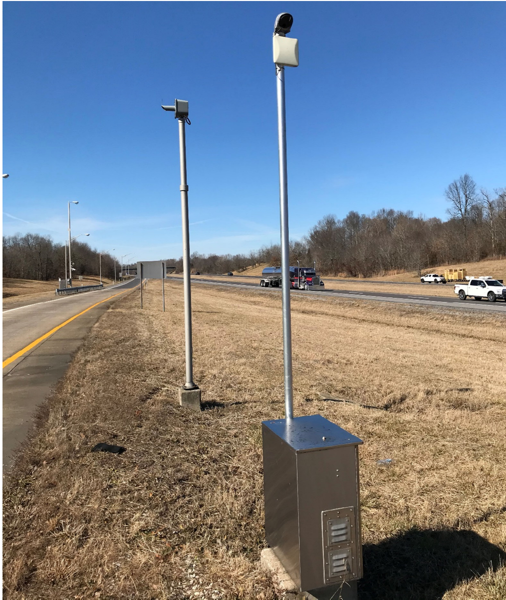
Figure 10. WIM and Height Detector Cabinet
