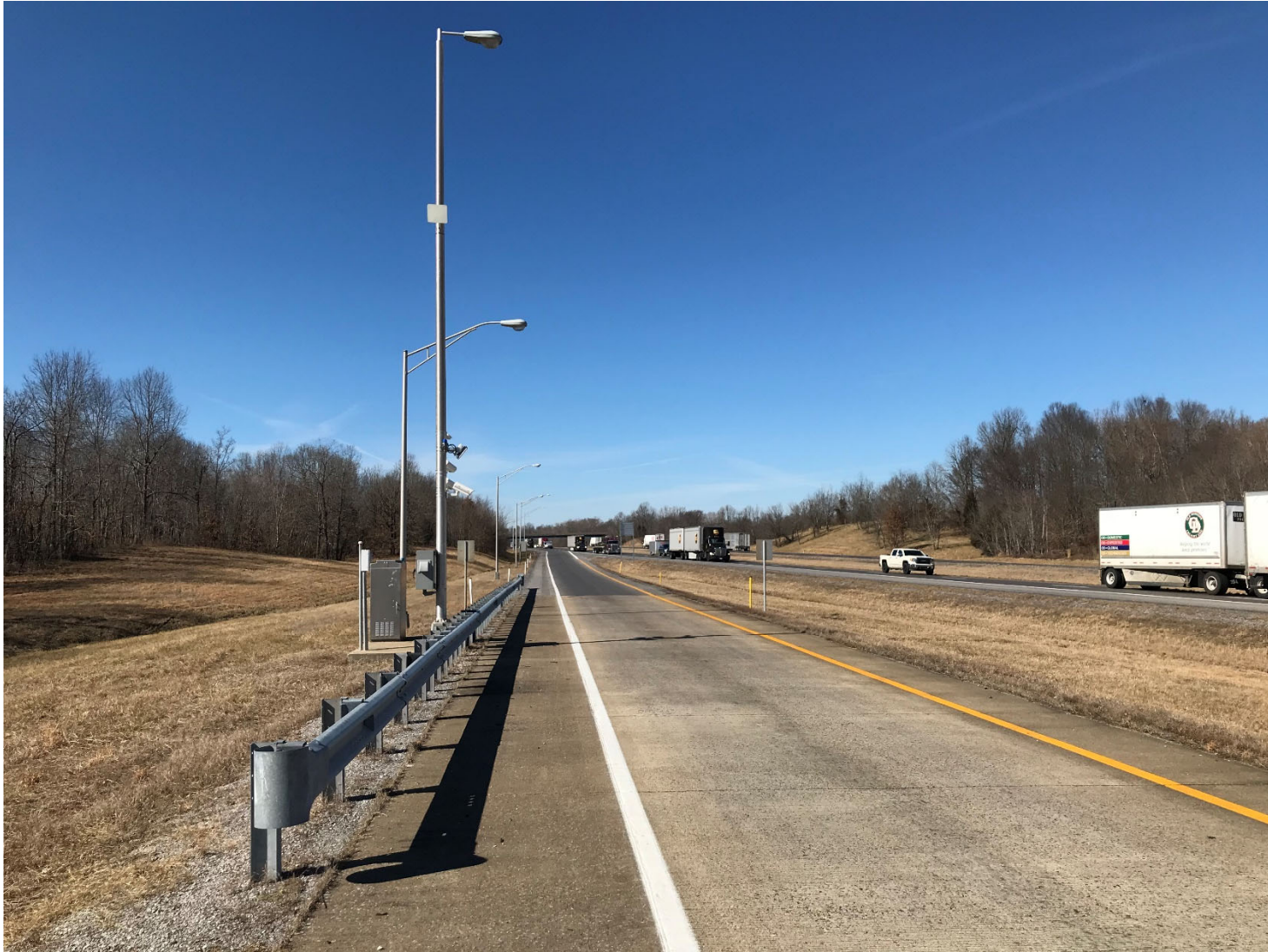
Figure 5. End Guardrail and KATS Camera Pole
