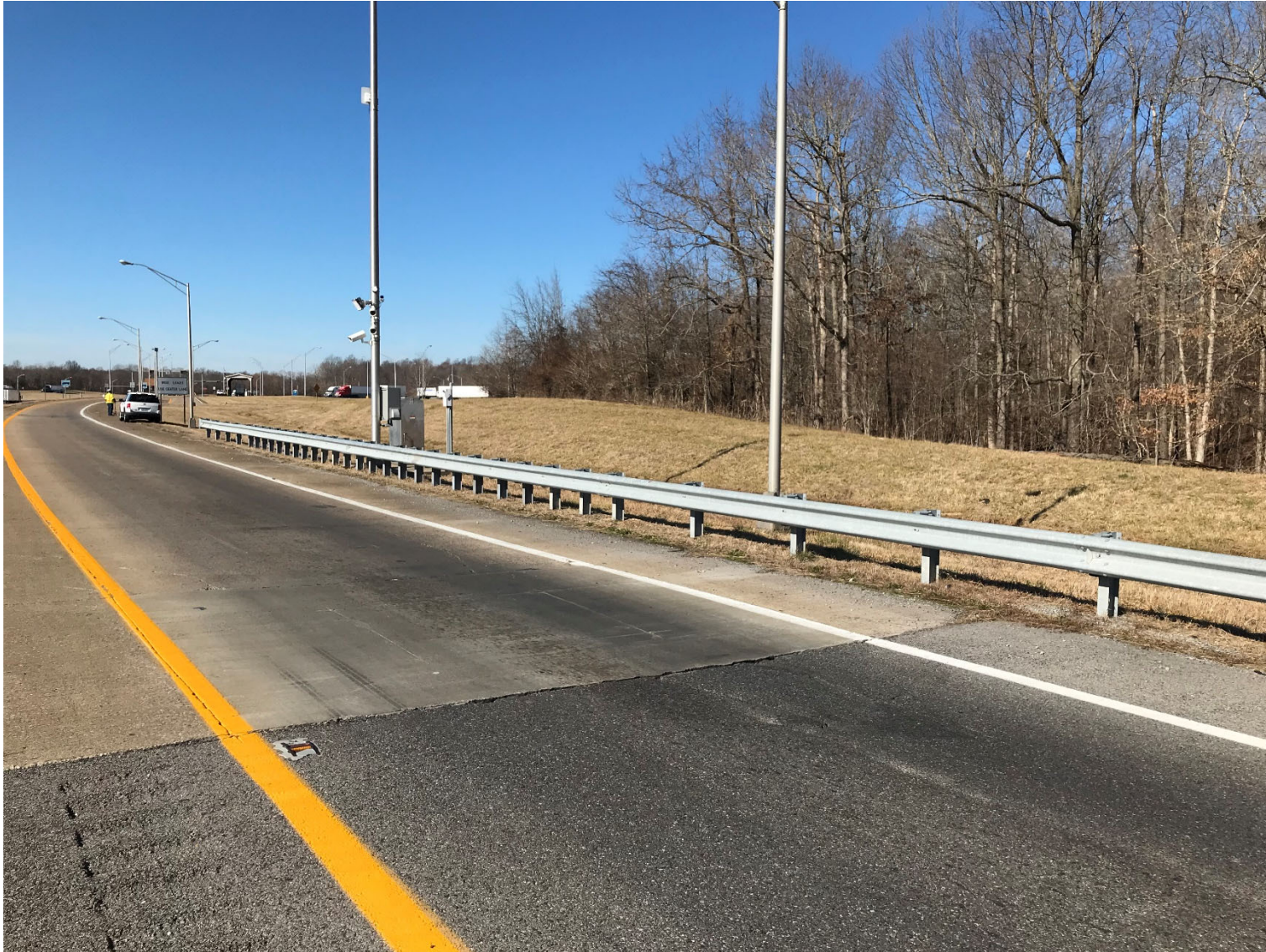
Figure 13. Start of Concrete and KATS Camera Pole
