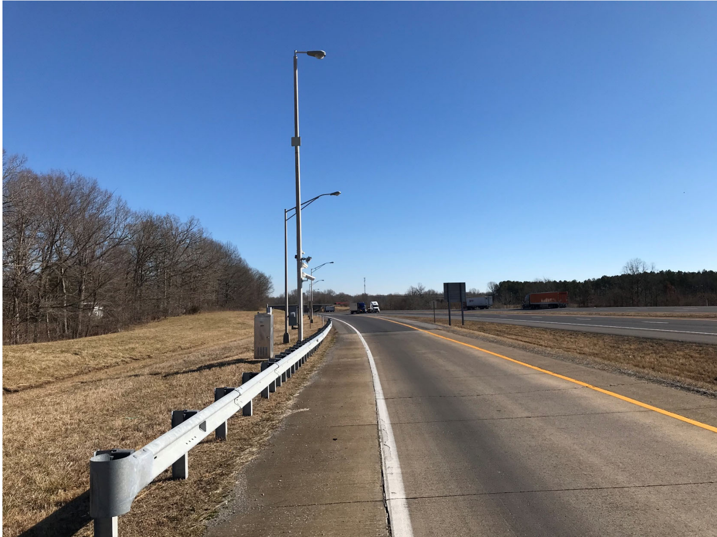
Figure 14. KATS Pole and Cabinet
