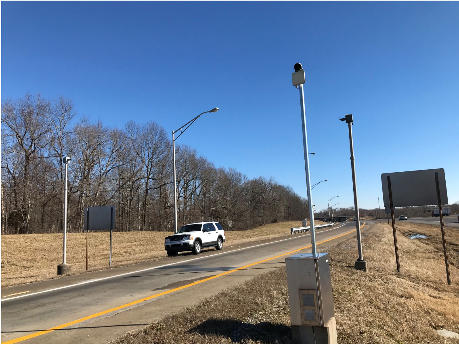
Figure 15. WIM and Height Detector/Cabinet
